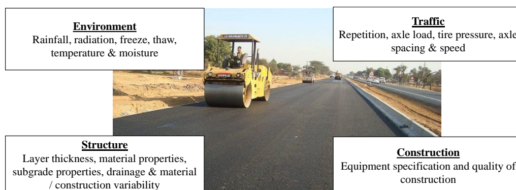
Figure 2: Factors Affecting Flexible Pavement Performance
