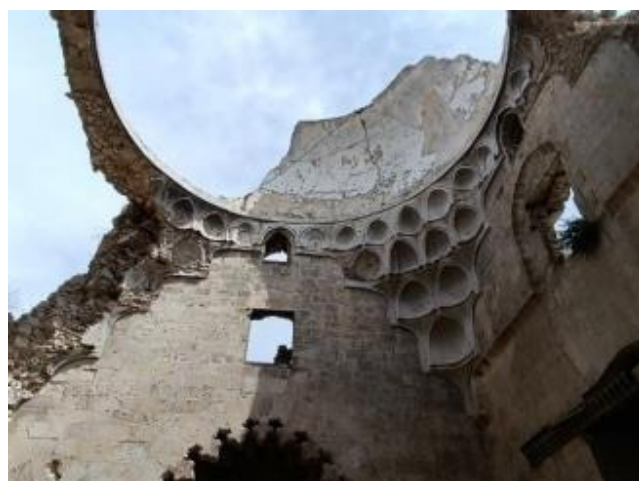
Figure 10. Increased deterioration in the dome of the great hall after the earthquake.
