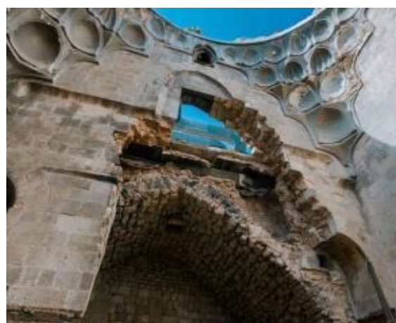
Figure 15. Partial collapse of the western wall of the large hall.
