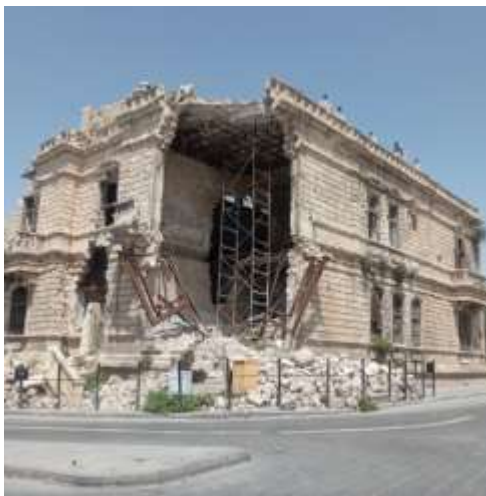
Figure 14: current condition of the building- Department of Immigration
