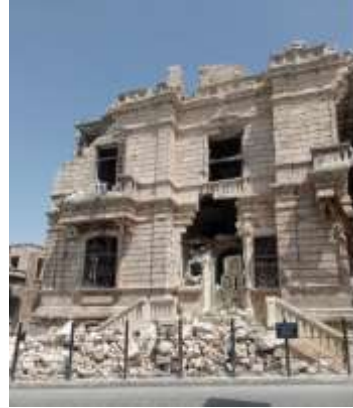
Figure 3: west façade with main entrance- Department of Immigration
