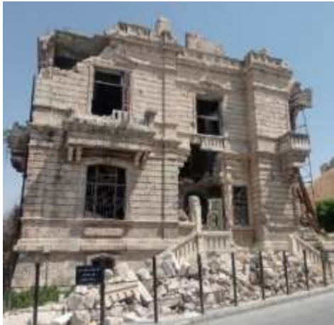
Figure 16: current condition of the building- Department of Immigration
